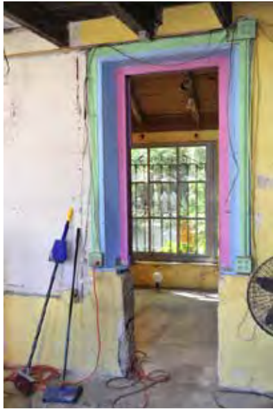
Figure 4. Converted window. Photo by Marla Holden, 2018.
