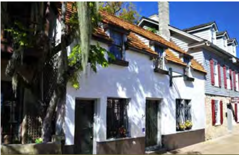
Figure 1. East (front) elevation of the Paredes-Dodge House and Rodriguez-Avero-Sanchez House to the north (right). Photo by Marla Holden, 2018.
